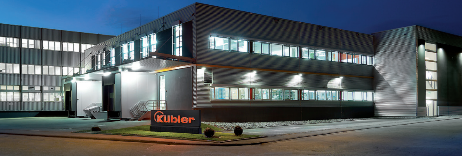
Kübler Headquarters, Villingen-Schwenningen, Germany
